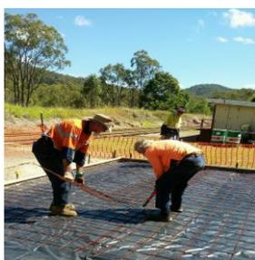
Dave, Terry and Keith are doing slab preparations for the Sleeper Cutter display and the M Series carriage cover near the Station building.
